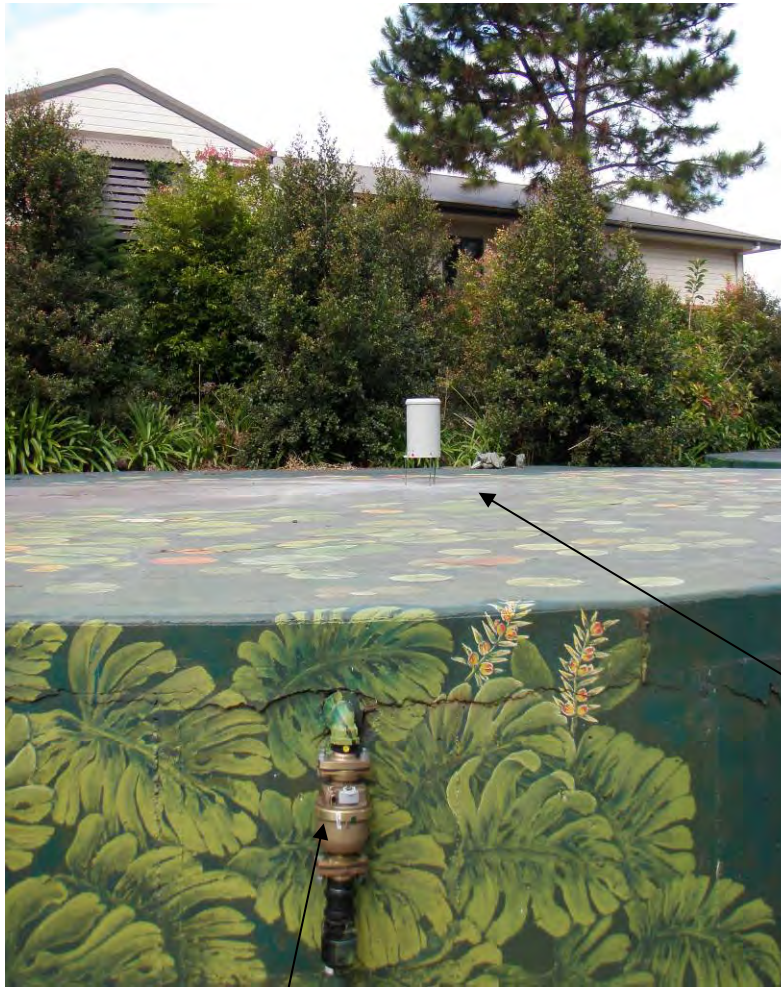
Meter for bore top-up
